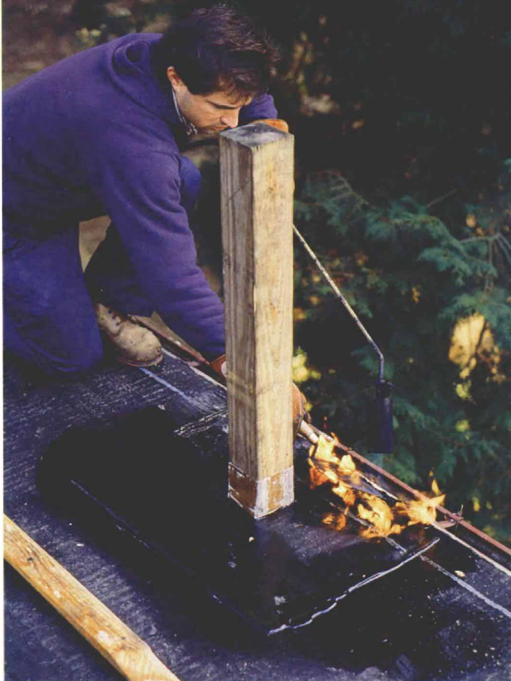
Fused flashings. One of the advantages of a single-ply modified-bitumen roof is that repairs and alterations can be heat-welded to the membrane long after the initial installation. Here, flashing strips of bitumen, which cover the copper base flashings around the 4x4 posts, are being fused to the roof membrane.
